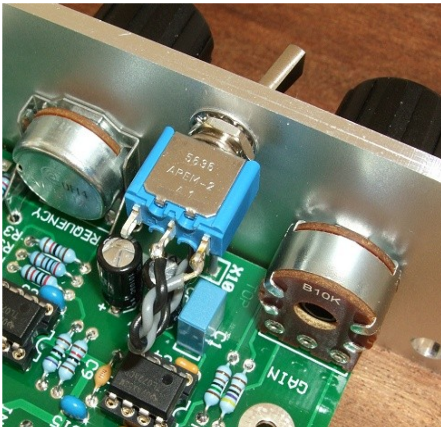
The standard EFG's 'x10' switch. Note that the twisted pair connects to the top pair of lugs on the switch.
