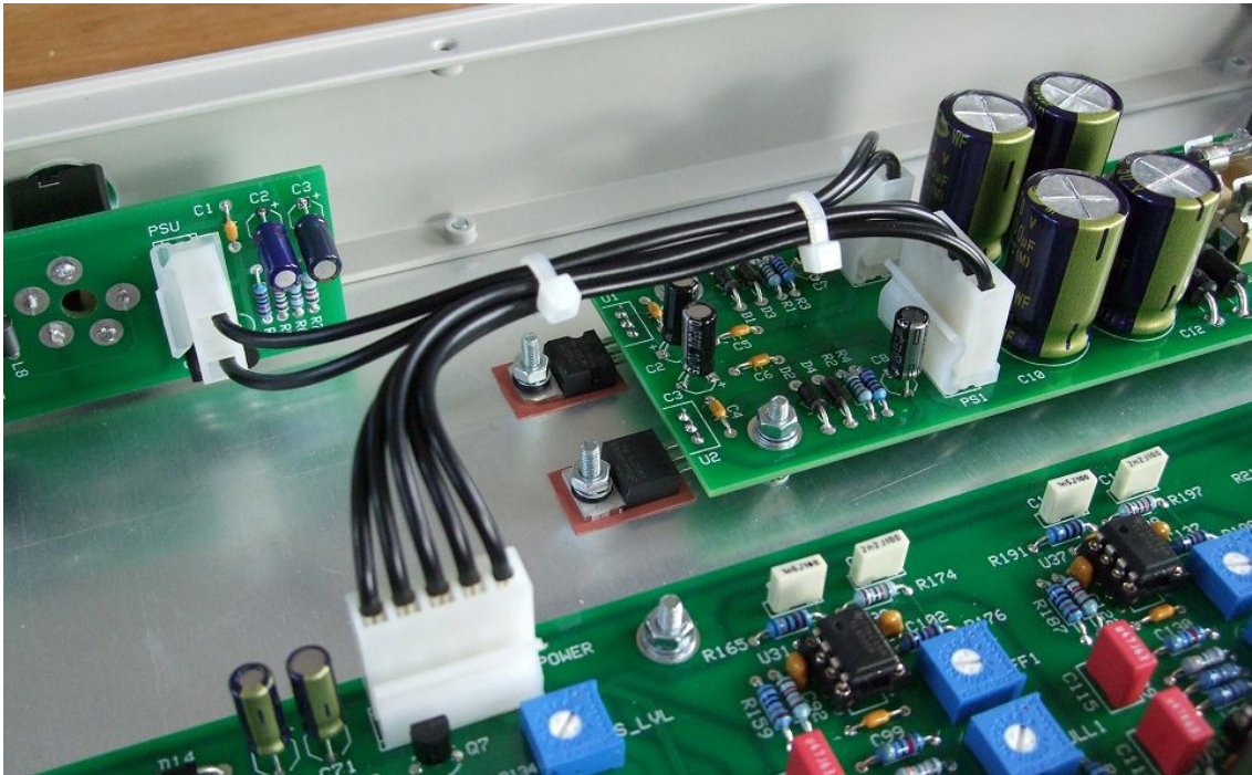
The power distribution within a SRE330. The five way interconnect carries +/-15V, 0V and case ground. The three way interconnect carries just +15V and 0V.
